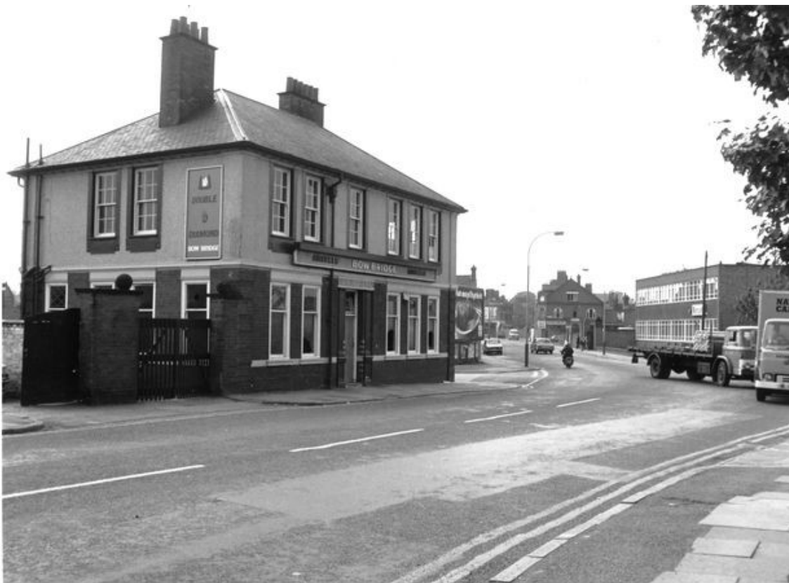
The Bow Bridge pub photographed by Graham Freer shortly before demolition
